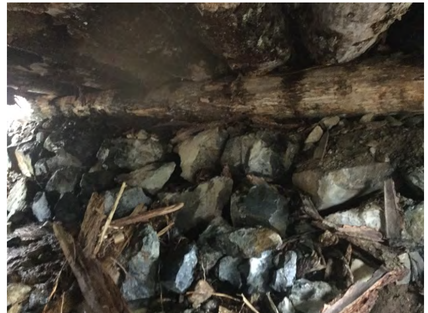
Left Bank Abutment when facing downstream
