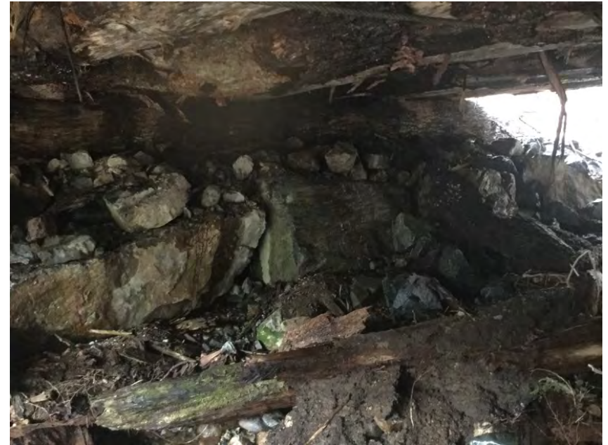
Right Bank Abutment when facing downstream
